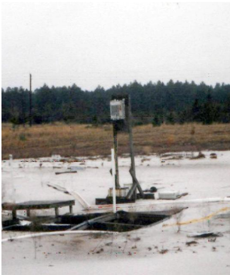
Fig. 5. An underground launcher
