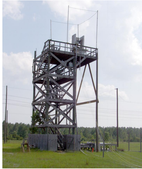
Fig. 2. A stationary 12-channel launcher in the form of a tower (a height of an upper tower landing is 11 m)
